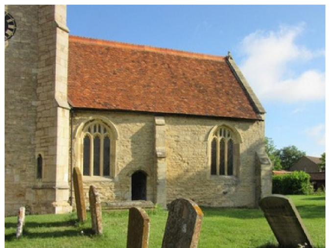
Handmade clay tiles on the roof of St Laud's.
