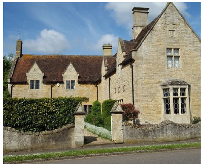
Home Farmhouse is of randomly coursed stone under plain tiles. The gables and dormers are coped with kneeler stones. The windows are lozenge patterned in metal.
