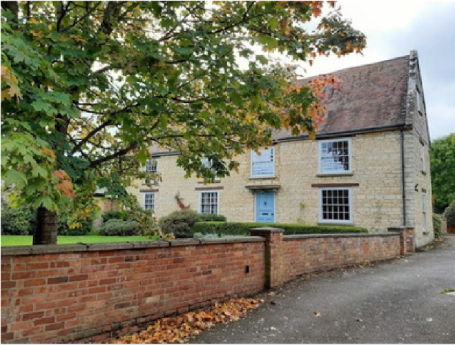
An elegant panel door at Bakers Farmhouse with 'eight over eight' pane vertically hung, flush fitting, sliding sash windows
