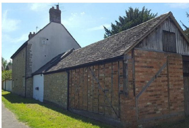
This outbuilding displays a variety of traditional building materials and methods
